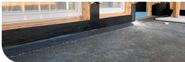
Waterproofing of OSB boarded CLT prefabricated balcony
